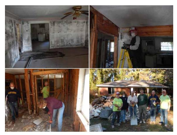
Top Left: View of the living room prior to demolition. Note mold stains on walls, damaged floor, and ceiling fan blades warped by moisture.
